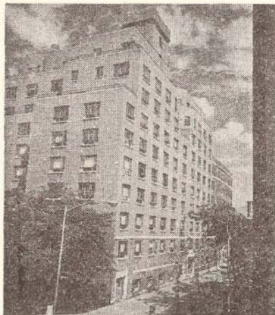
Brooklyn Bethel home constructed in 1950, showing 1927 structure on far end and 1969 building in foreground at right
