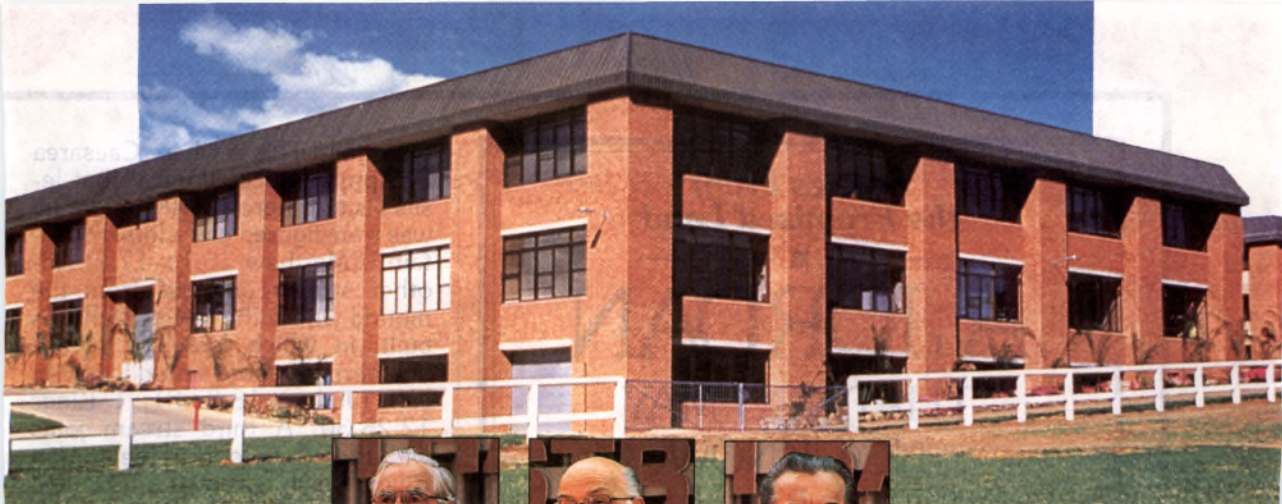
New addition to Watch Tower printery at Ingleburn, N.S.W., Australia
