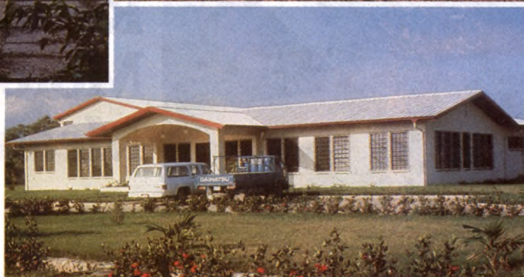
Views of the Assembly Hall (top right) and of the new branch
