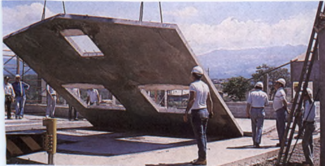
A precast wall section being tilted up . . . and set in place
