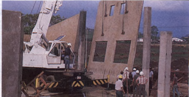
A precast wall section being tilted up . . . and set in place
