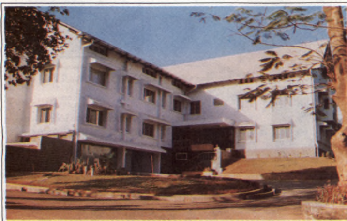
New branch headquarters south of Bombay
