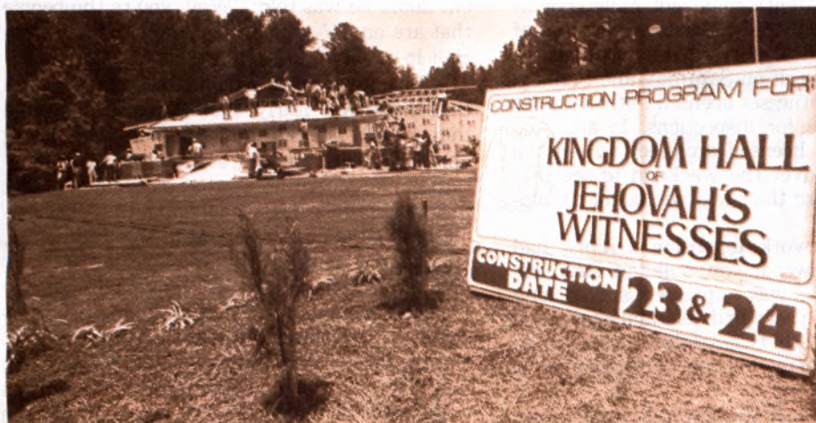
With a crew like this a Kingdom Hall can be built in two days
