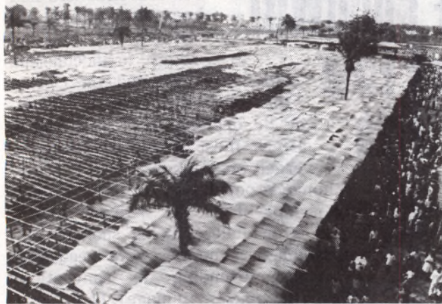
Roofing of the assembly pavilions in progress at Lagos, Nigeria
