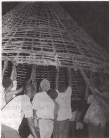
Building assembly facilities in Sierra Leone
