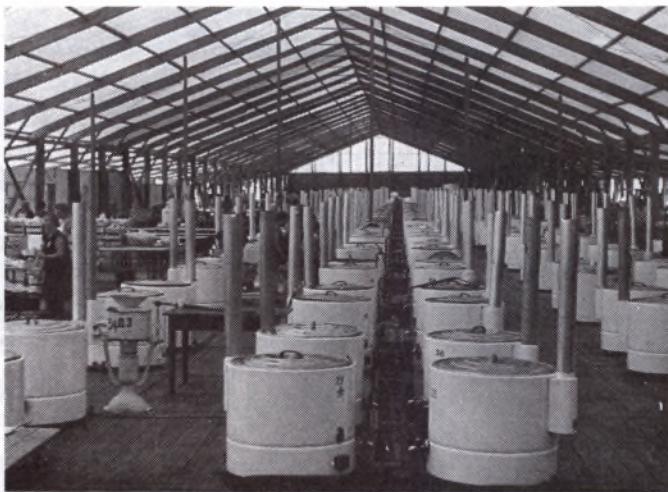
Section of huge kitchen at Nuremberg showing some of dozens of steam cookers used in preparing meals
