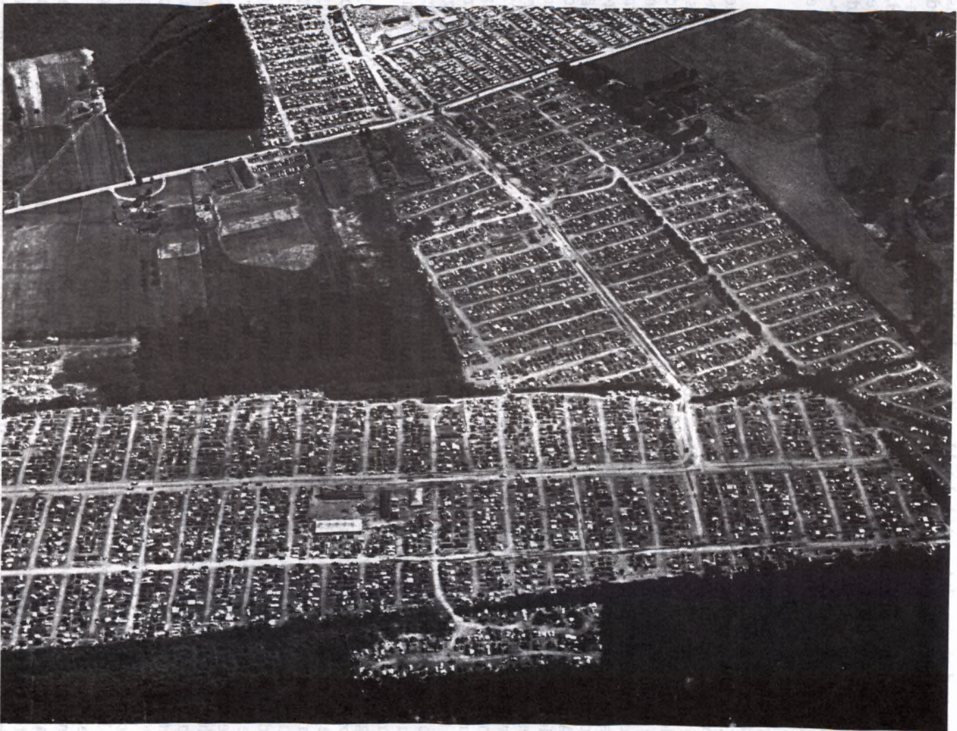
Aerial view of part of Trailer City
