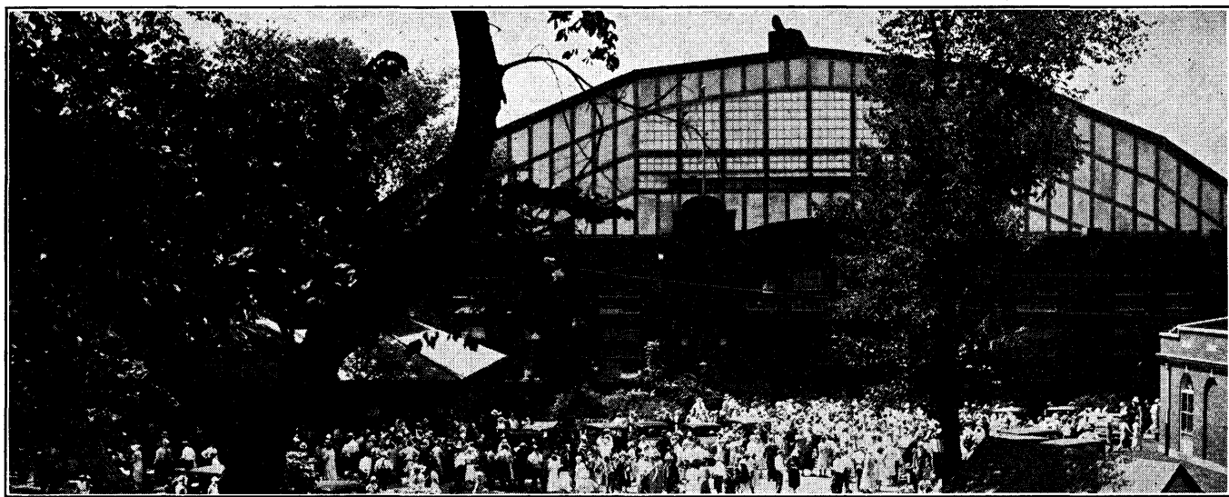
The Thousands That Could Not Get Into the Coliseum Were Accommodated in the Grandstand, Dining Room, and on the Grounds, Whither the Public Address System Carried Judge Rutherford's Voice.
