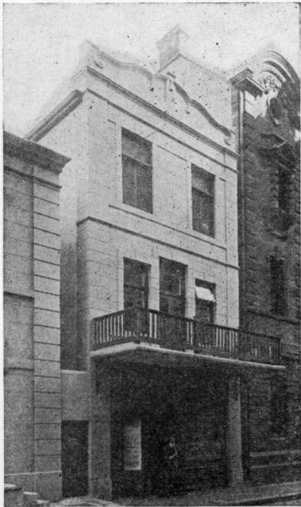
Bethel Home and Office in Cape Town.
