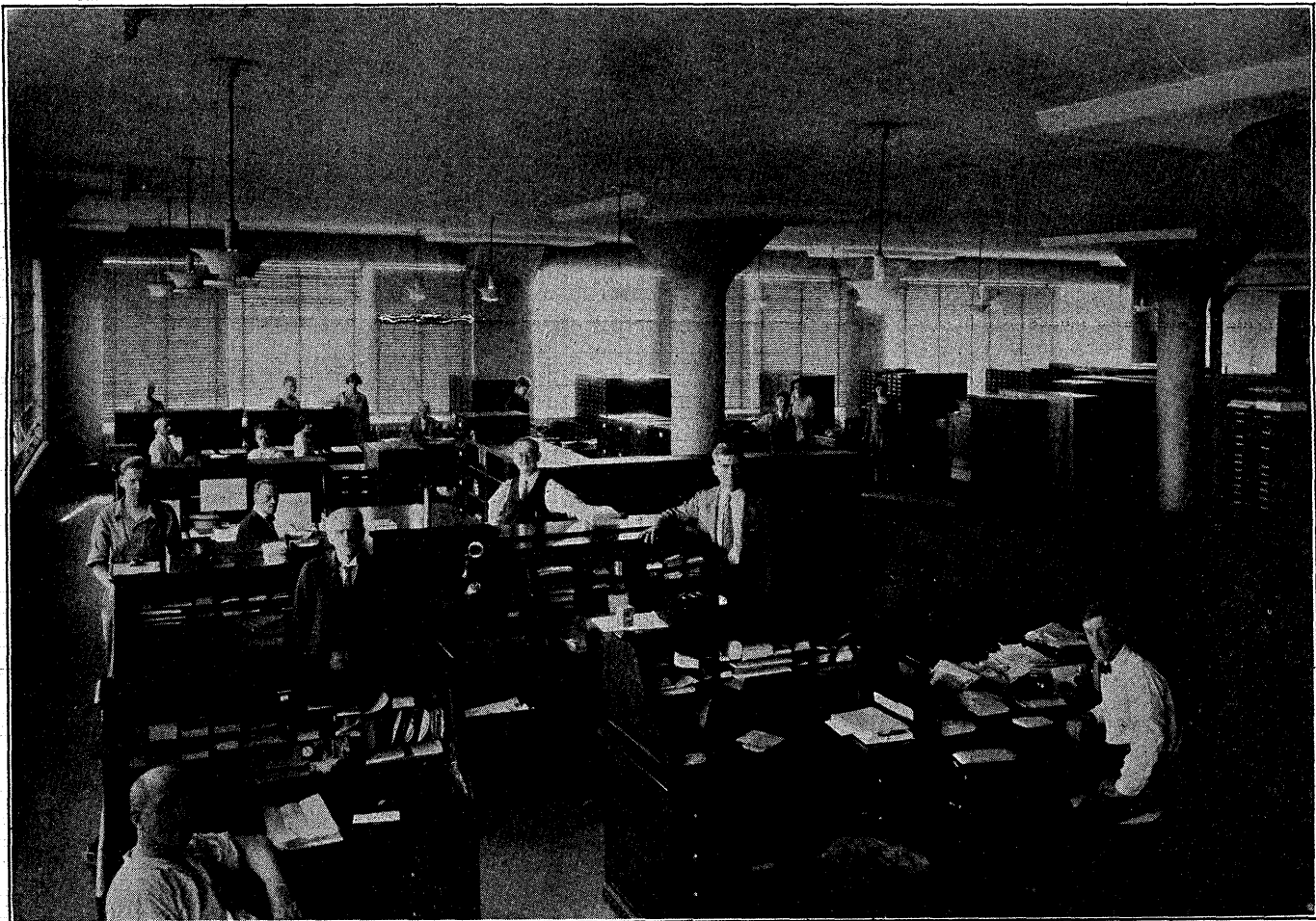
Northeast Corner of General Office—Eighth Floor
