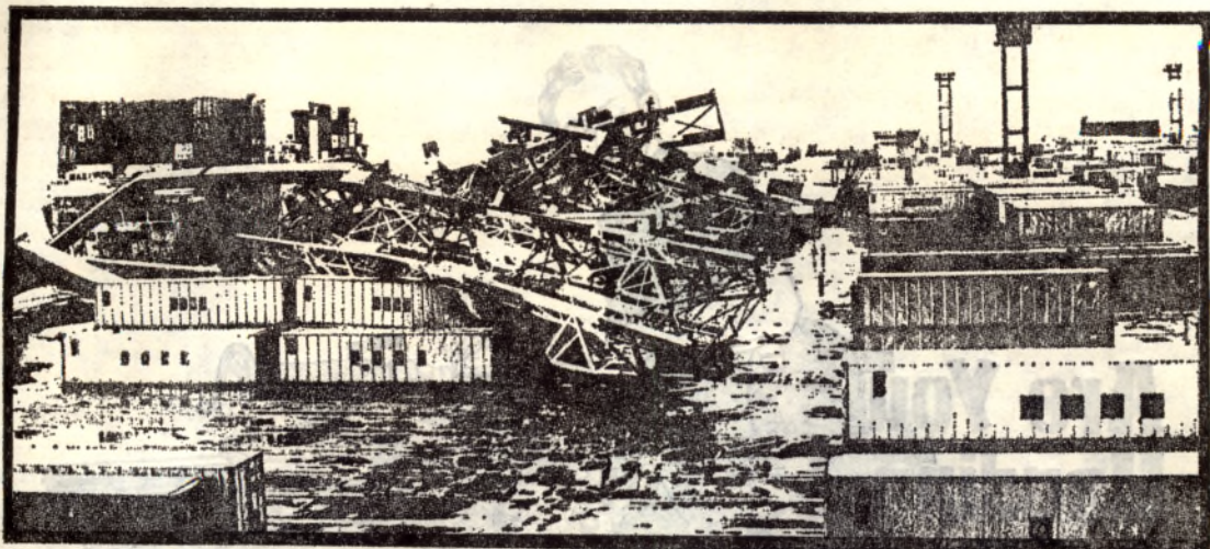
Damage wreaked by Typhoon Thelma in the Kaohsiung harbor area
