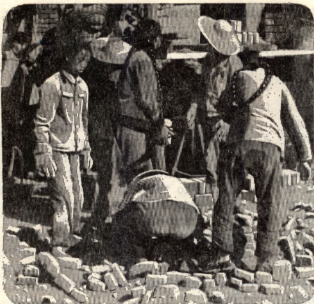
Women labor to repair earthquake damage in Peking
