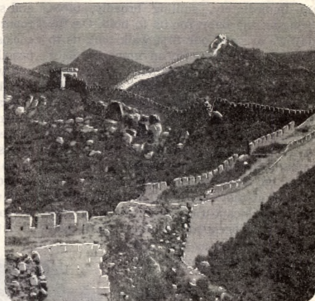
This portion of the Great Wall shows the collapse of unmaintained sections
