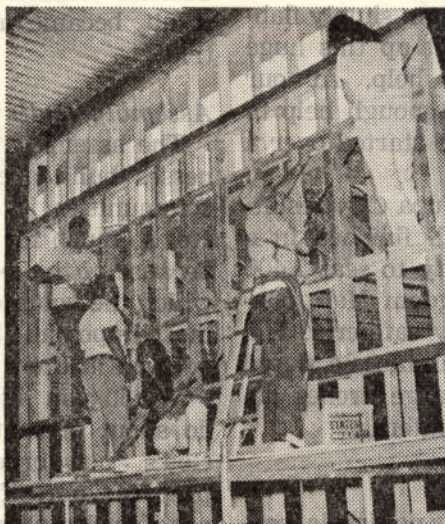
Construction of Yuba City, California, assembly hall by volunteer workers
