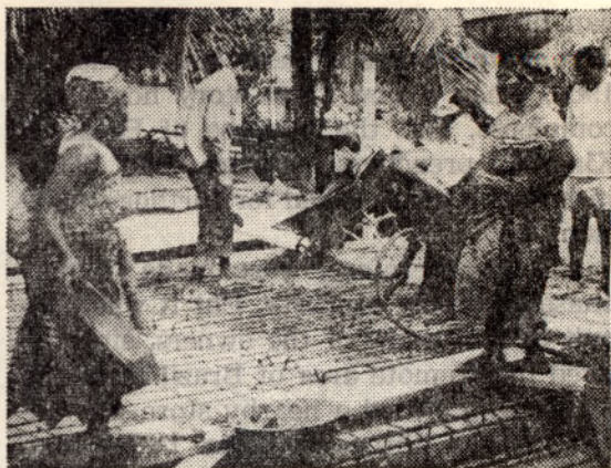
A new factory for printing Bible literature has been completed in Ghana; here both men and women, all volunteers, share in pouring the concrete
