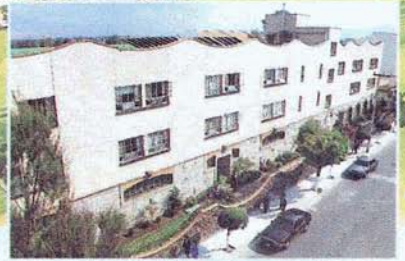
Office facilities being used in 1992
