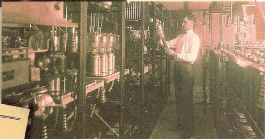
Broadcasting equipment at station WORD, near Chicago, Illinois; owned and operated by the Society
