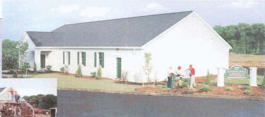
Major work completed, Sunday, 6:10 p.m.
